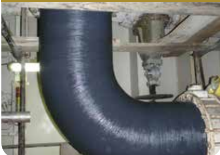
Pipe repair & reinforcement
