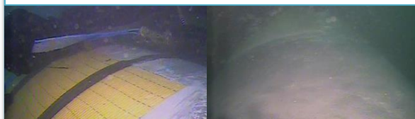
Composite plates fixing & second primer application (steps 2 & 3)
