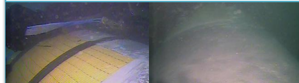
Composite plates fixing & second primer application (steps 2 & 3)
