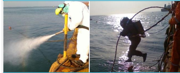
Surface preparation / Sandblasting
