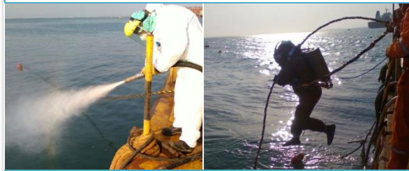
Surface preparation / Sandblasting
