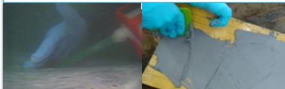
Primer & composite plates with filler applications (steps 1 & 2)
