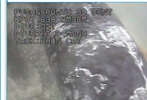
Pipe before surface preparation
