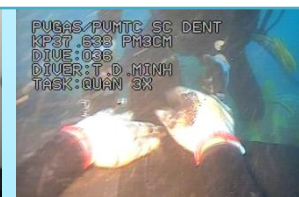
Tape impregnation using BOBIPREG & R4D-S wrapping (step 4)
