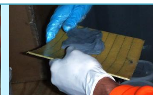
Primer & composite plate with filler application (steps 1 & 2)
