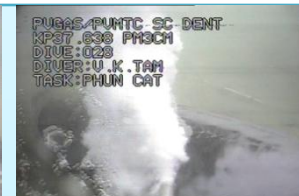
Sandblasting in progress
