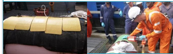
Composite plate manufacture on the foot print of the dented area & primer application (training picture).
