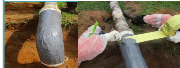
Mastic application and wrapping process with Kevlar® tape and resin
