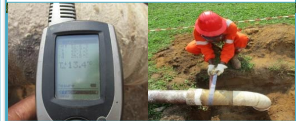
Climatic conditions measurements and surface preparation
