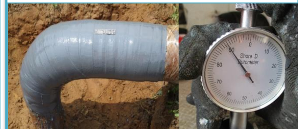
View of the repair completed and hardness measurements
