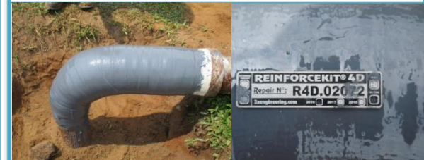
View of the elbow after wrapping and id plate positioning
